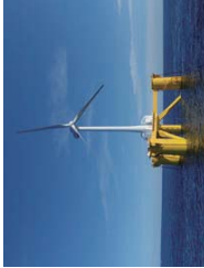
A 7-megawatt floating wind turbine has been constructed off the coast of Fukushima under a project commissioned by the Ministry of Economy, Trade and Industry. The blades reach a height of 200 meters (about 660 feet) above the ocean. Photo: Fukushima Offshore Wind Consortium.
