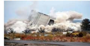
Deactivate, decontaminate, decommission and demolish facilities (401 of 522 to date)
