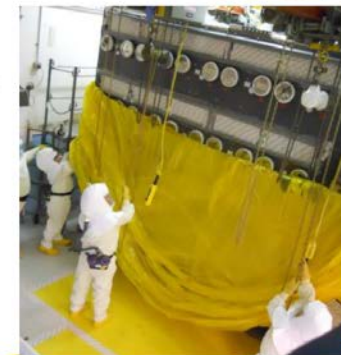
Removed 204 of 238 glove-boxes as to date from highest-hazard facility at Hanford, the Plutonium Finishing Plant.
