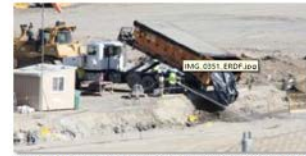
Treat, transport and dispose of waste debris at Hanford's disposal facility (15.5 million tons disposed to date)
