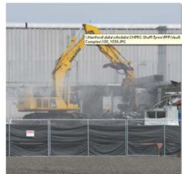
Demolished plutonium vaults - 55 of 81 Plutonium Finishing Plant facilities demolished to date
